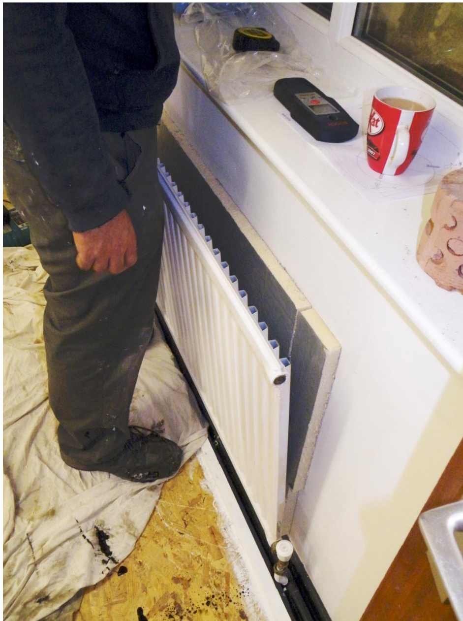
Insulation installed behind radiators
